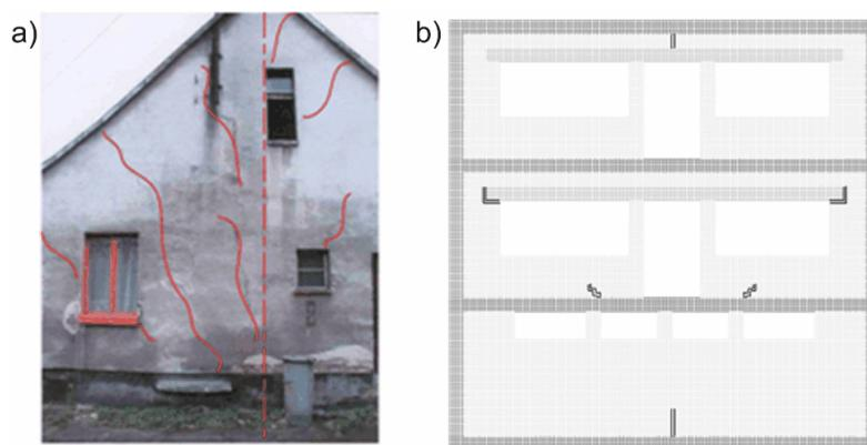
**Fig. 1.** Typical damage of the building caused by a convex basin (NW): a) real building, b) numerical model
