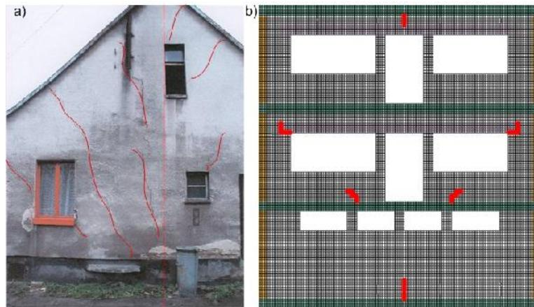
Figure 3: Cracks set into the wall: a) real photo, b) numerical model
