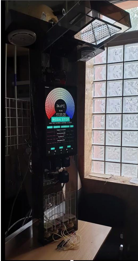
Fig. 7a. General view.
